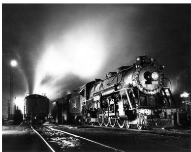
NdeM, Valley of Mexico engine terminal, Tlalnepantla, 1960
